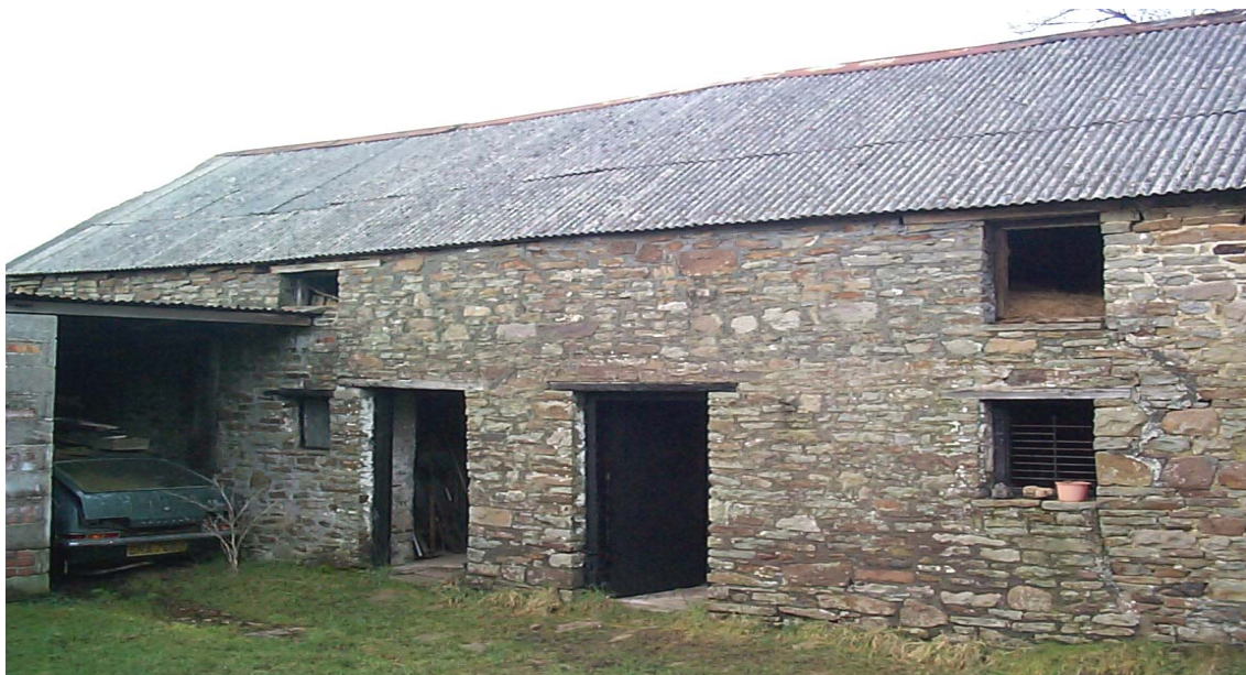
Ty'n-y-waun, Heol-y-Cyw (4227M); hearth-passage house with later alterations. It became an outbuilding when a new farmhouse was built in the 1840s.
